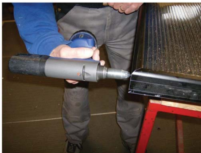
20. New pop rivets are put in the end gable.
