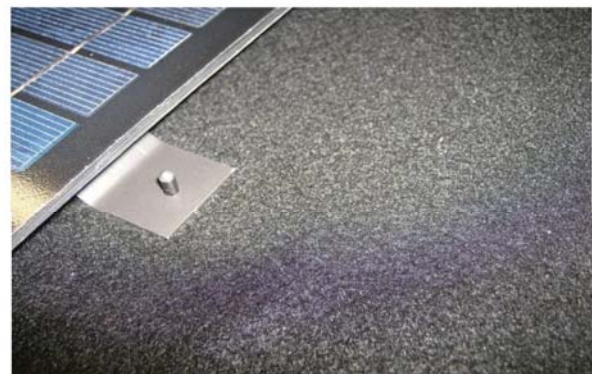
17. The pop rivet has to catch the bracket/fitting of the solar cell.
